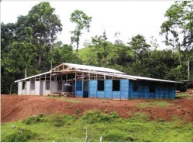
The Ministry Center under construction
